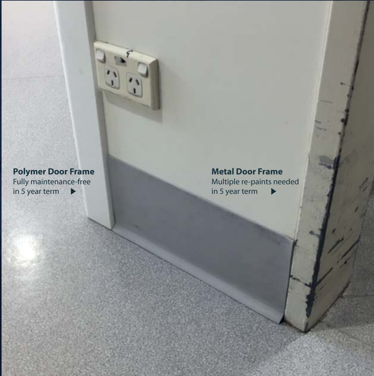
Polymer Door Frame (LEFT) vs Conventional Metal Door Frames (RIGHT) after 5 Years
